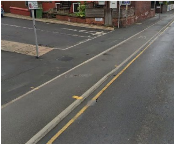
Figure 6: an entry treatment of both a stepped cycle track and continuous footway (Google Maps)
